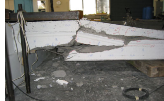
Negative Moment Failure (NMF)
