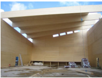
CLT On Edge – Long Span Roof Beams
