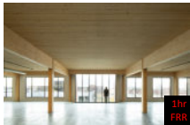
Type IV - T3, Minneapolis MN 6-Story wood over 1 Story Concrete <85ft, Exposed Wood 1hr FRR
