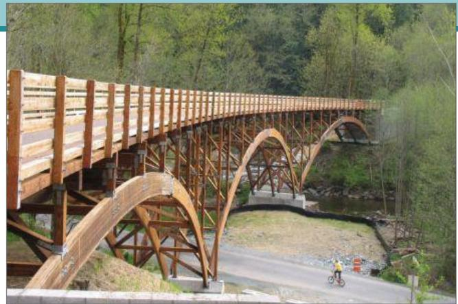
sure-treatment results in preservatives penetrating 3/4" into the side grain and up to 6" in the end grain of each member.
