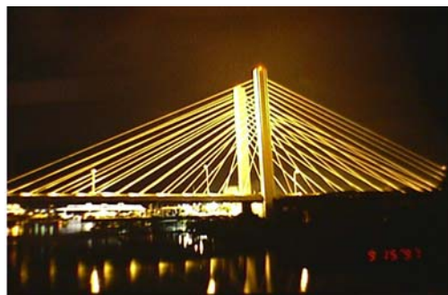
Foss Waterway Cable-Stayed Bridge -1997
