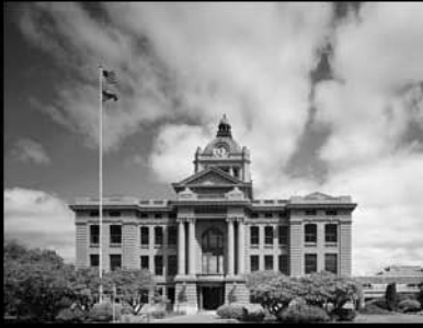
Grays Harbor County Courthouse Renovation
