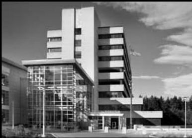
Naval Hospital Bremerton Seismic Upgrades
