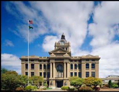
Grays Harbor County Courthouse Renovation
