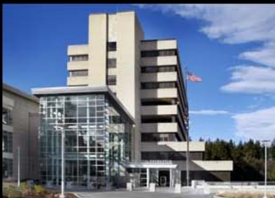
Naval Hospital Bremerton Seismic Upgrades
