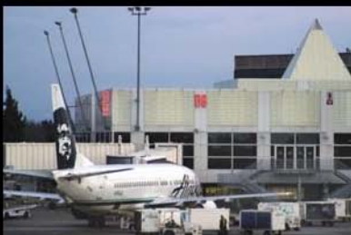
SeaTac Airport Seismic Improvements Program
