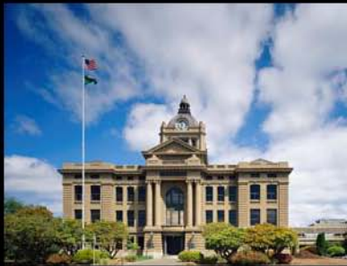
Grays Harbor County Courthouse Renovation
