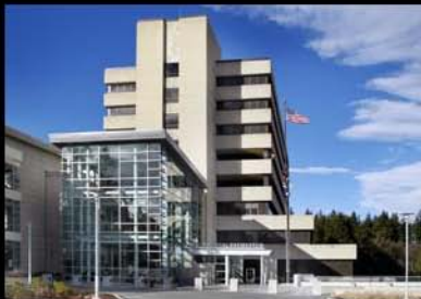
Naval Hospital Bremerton Seismic Upgrades
