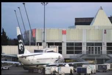
SeaTac Airport Seismic Improvements Program
